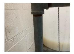
• Lead lines are gray or silver in color. Lead is a soft metal and can easily be scratched. Lead lines are <u>NOT</u> magnetic.
