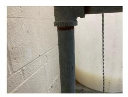
Lead lines are gray or silver in color. Lead is a soft metal and can easily be scratched.
